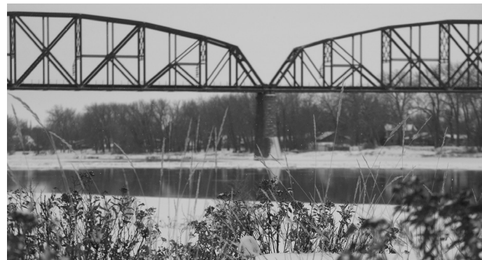
The BNSF bridge crosses from Bismarck to Mandan. (Credit: Zachary Weiland)
